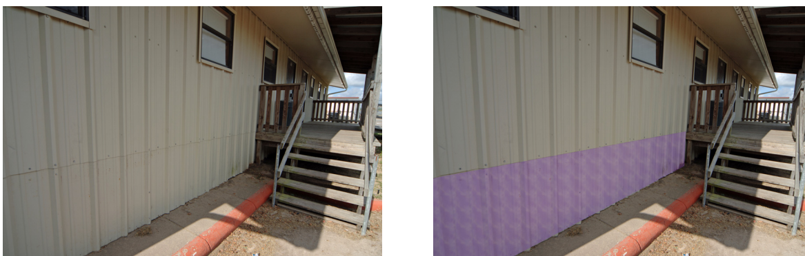
Figure 19.2 Extend siding to the ground (or screen spaces underneath) to prevent access to relocatable/portable buildings.
